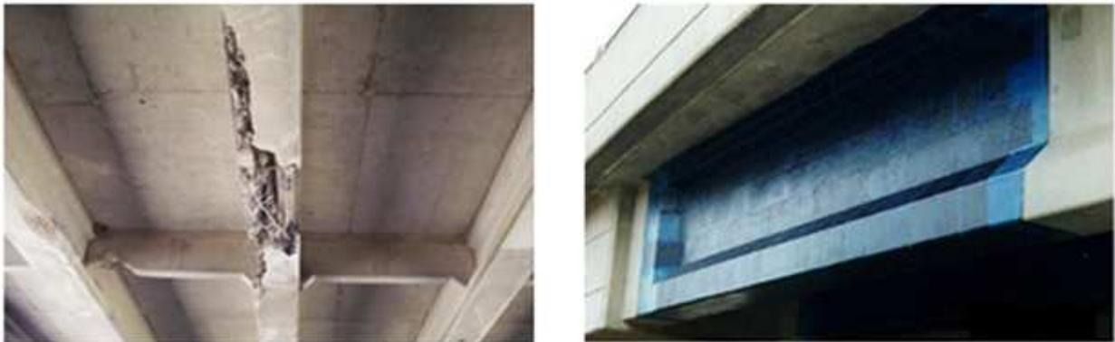
Fig. 1 Damaged and Strengthened Girders
