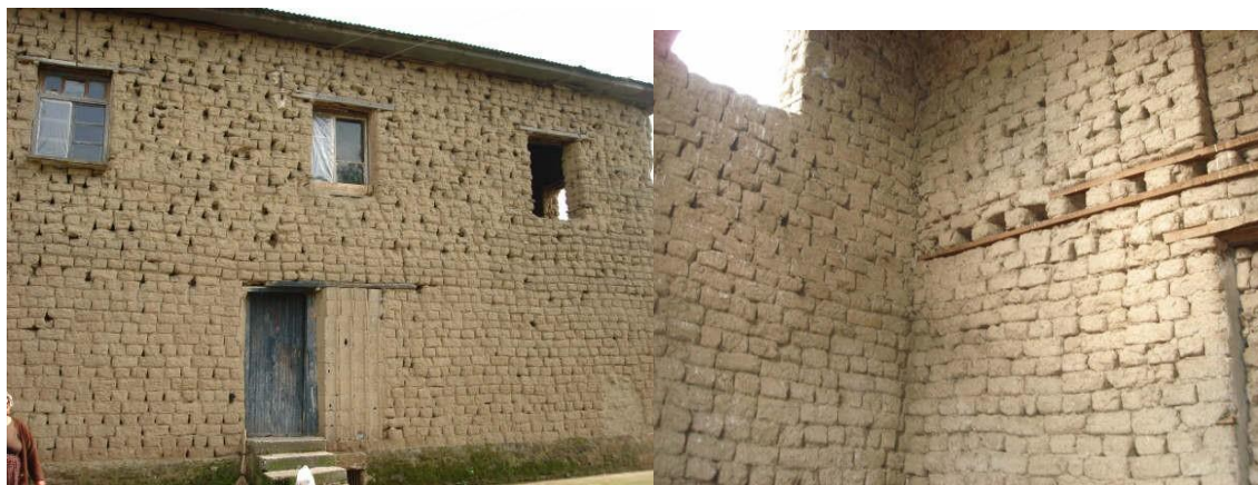
Fig. 10 Traditional mud brick house in Osmaniye
